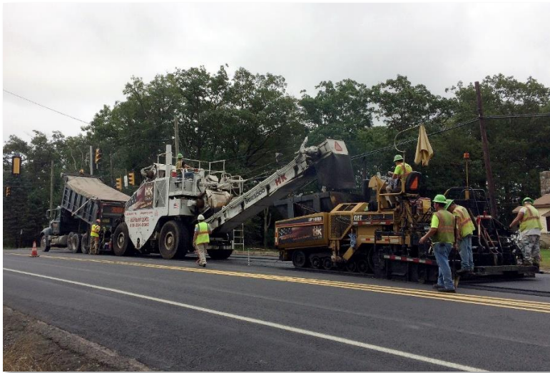
Pikes Creek Site Contractors performs paving maintenance on SR 11 (Photo 1 of 2)
