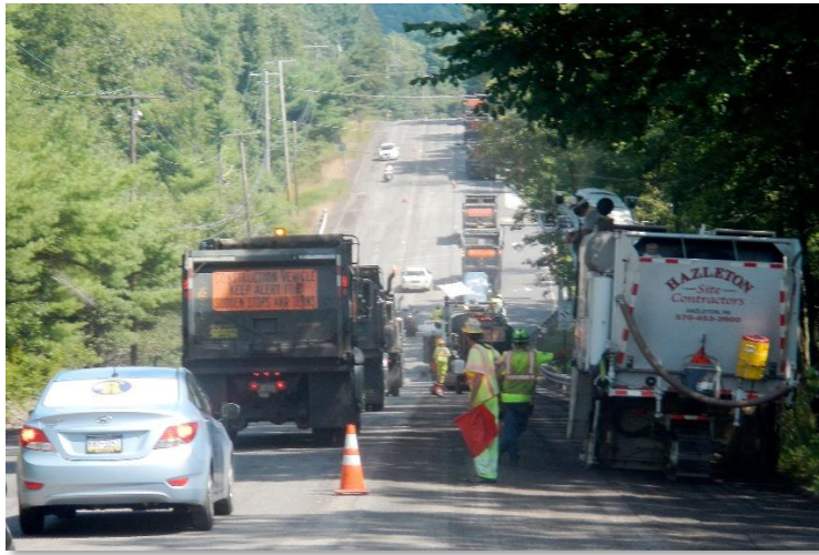
Pikes Creek Site Contractors performs paving maintenance on SR 11 (Photo 2 of 2)
