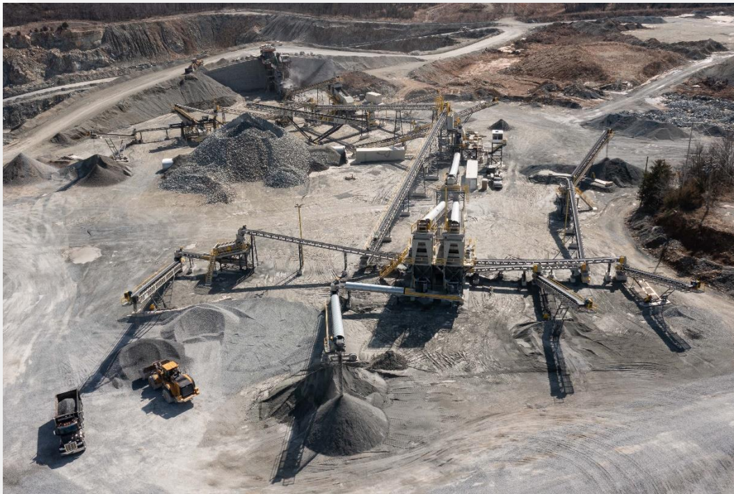
An aerial photo shows the entirely new and redesigned crushing plant at H&K's Penn/MD Quarry located in Peach Bottom, PA.
