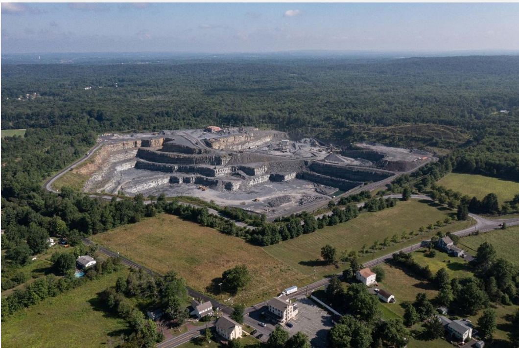
An aerial view of the H&K's Naceville Quarry located in Sellersville, PA.
